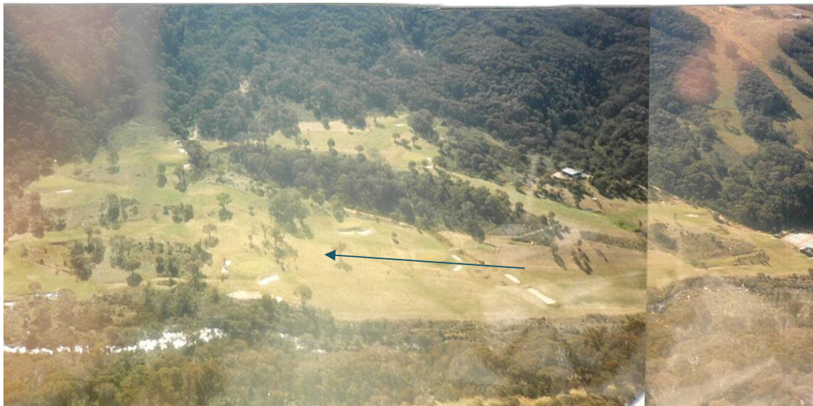
Plate 28. View north – arrow indicates approximate area of PAD. Photo date circa 1970s following construction.
